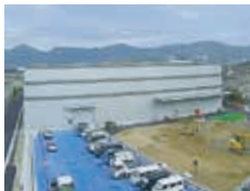
3rd machinery plant, under construction
